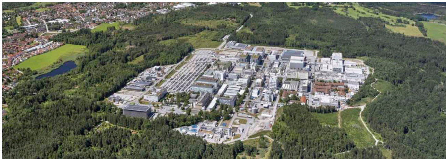
Biotechnologické centrum Roche Diagnostics, zdroj: https://www.roche.com/innovation/structure/rnd-locations/dia-penzberg
